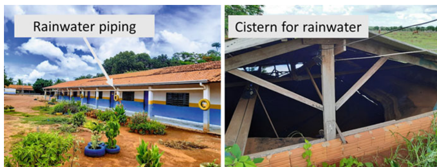
Fig. 12 Rainwater collection in rural school as an alternative to reduce stress due to lack of water. Source: authors
